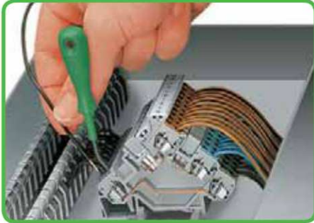
Conductor termination using an angled screwdriver (3.5 x 0.5) mm / (0.137 x 0.020) in.
