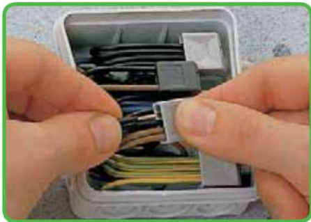
Connection: Insert stripped conductor fully!
