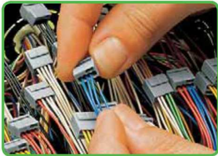
Termination: Insert stripped conductor fully.
