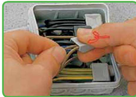
Removal: Hold wire to be removed and twist alternately left and right while pulling the conductor
