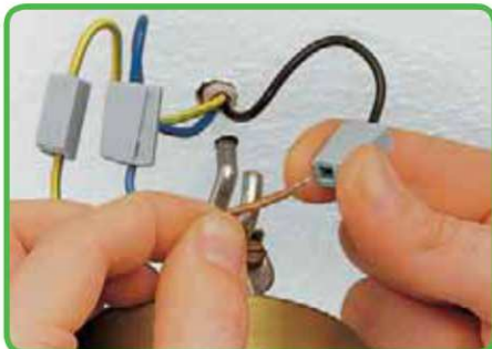
Lighting side terminations: Press button fully and insert stripped conductor into square entry and release.
