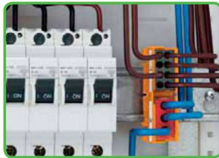
FIXED IN POSITION – on a DIN 35 rail (Mounting carrier series 773)
