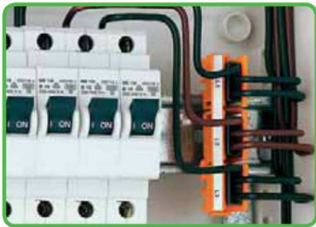
FIXED IN POSITION – on a DIN 35 rail (Mounting carrier series 273)
